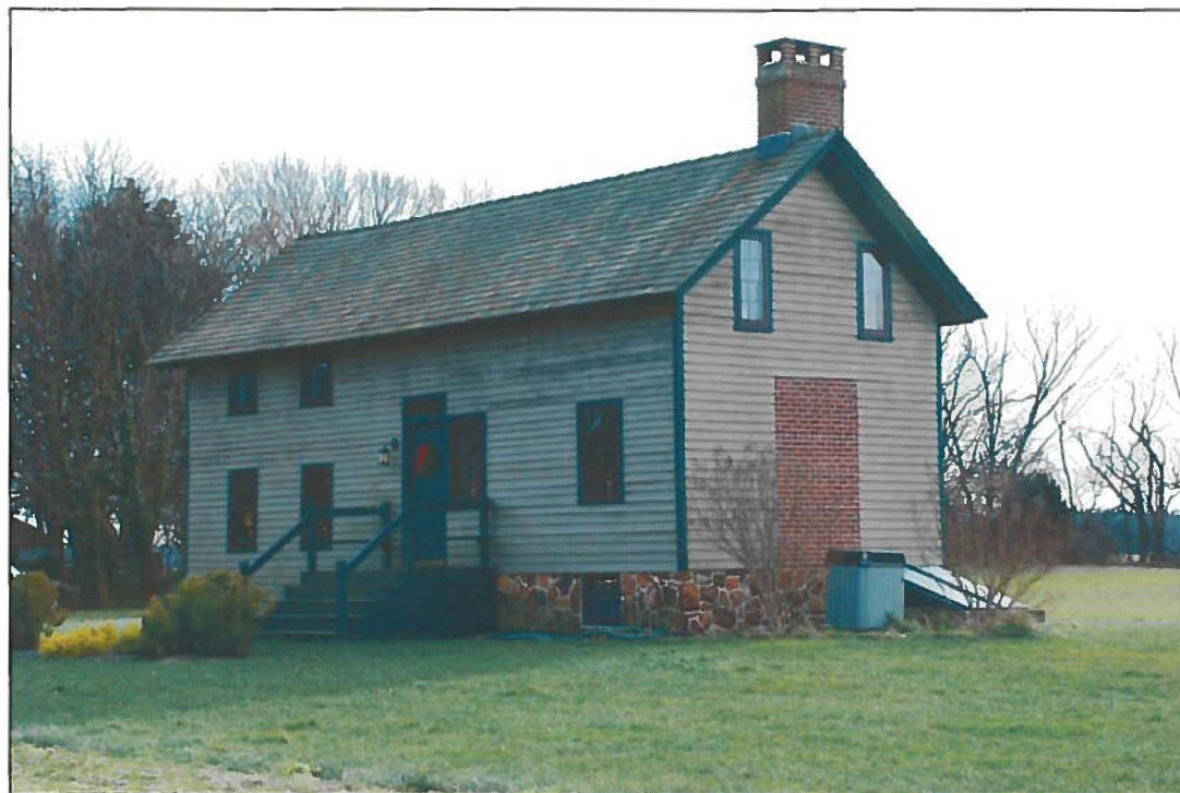
Figure 23: Charles Briggs House, Greenwich, a Hall-Plan, H-Bent Framed House. Built 1789. Left-Hand Section Added Circa 1850.
