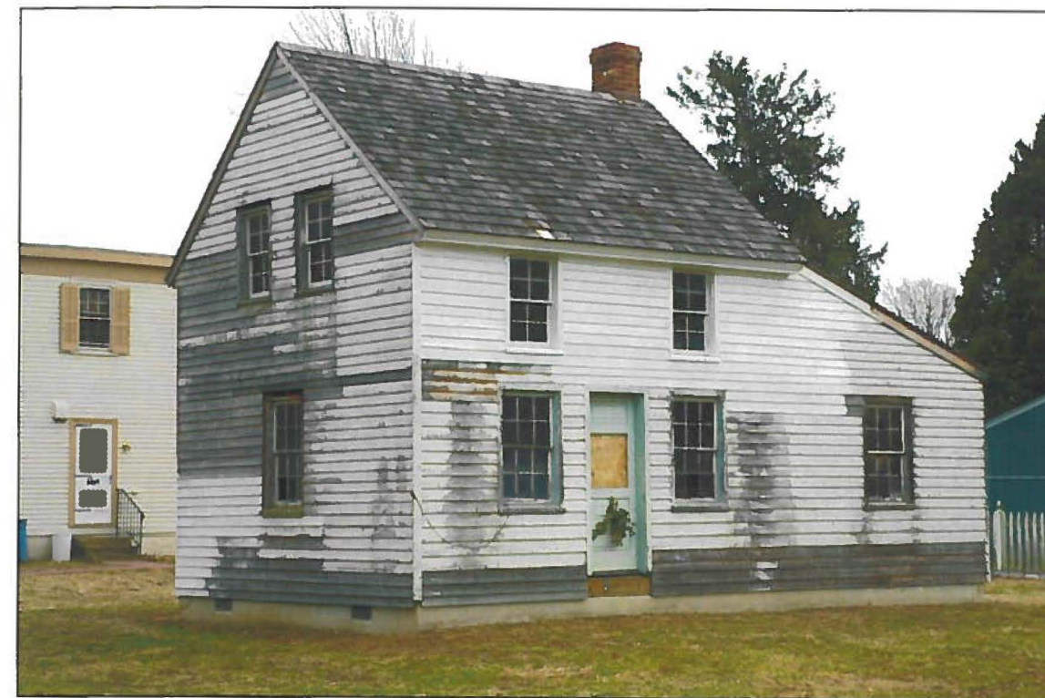
Figure 25: H-Bent Framed, Hall-Plan House in Mauricetown, Built Circa 1830.
