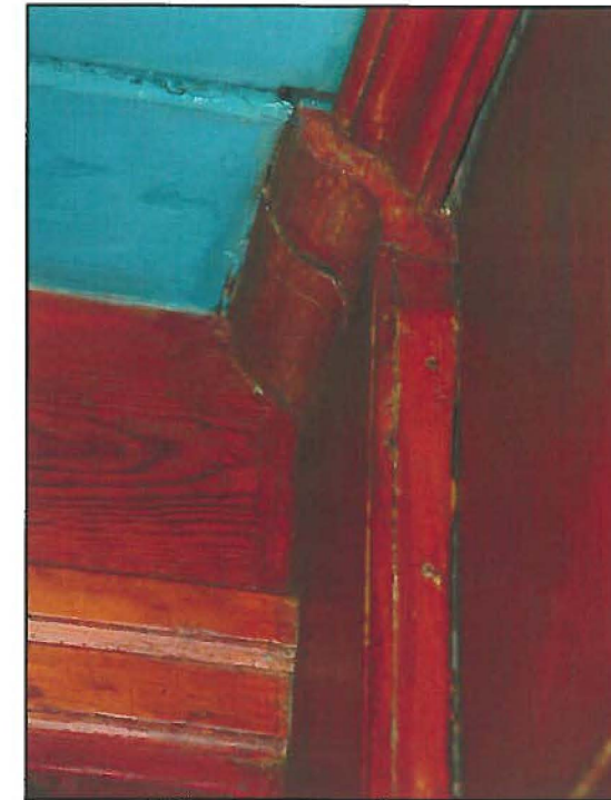
Figure 10: Shivers House Carved Cyma Reversa Post Capital at Story Post (Middle of Gable End), Under Summer Beam Supporting Second Floor. Post is Cased in Half-Inch Beaded Boards.
