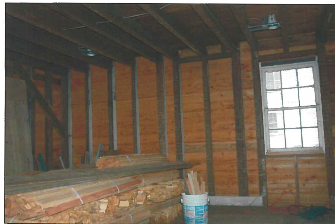
Figure 26: Interior of the Mauricetown House Showing Closely Spaced H-Bents.
