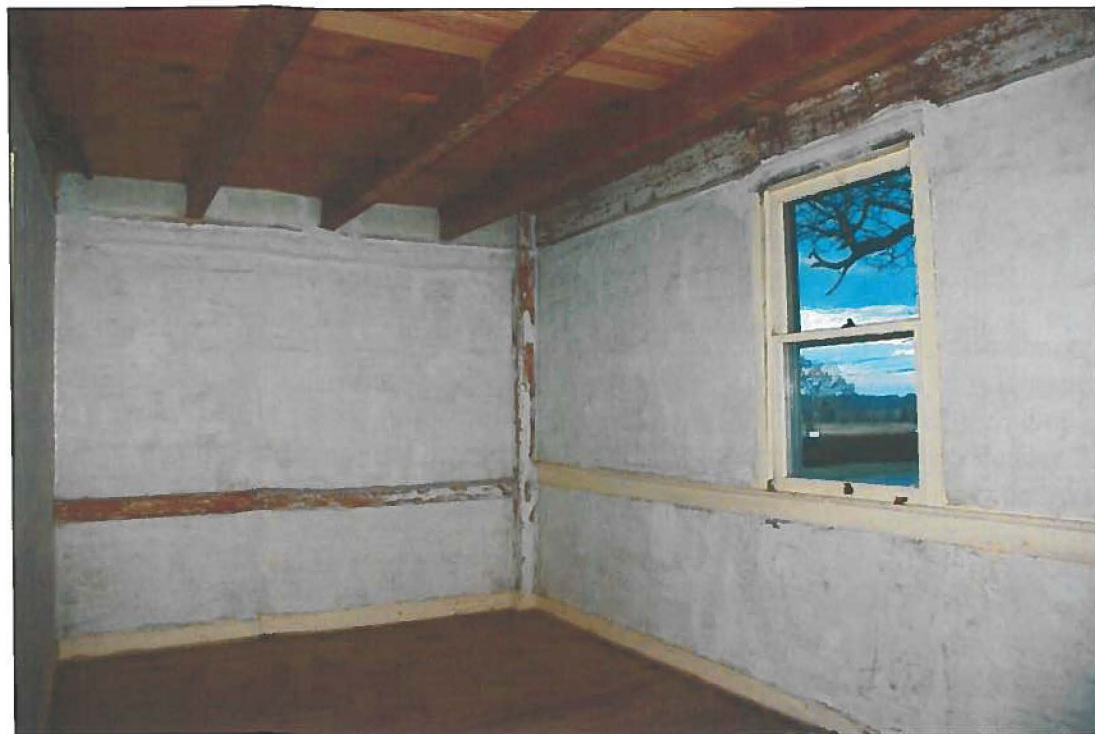
Figure 15: Watson House Second Floor Room Showing Articulated, Beaded-Cased Posts and Dressed, Chamfered Joists. Lath and Plaster was a Later Alteration Since Removed.
