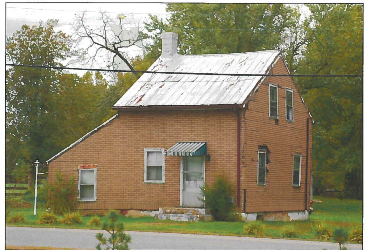
Figure 20: Abraham Richman House, Avis Mill, Pilesgrove Township, a One-And-One-Half Story, Double-Pile, Hall and Parlor-Plan, H-Bent-Framed House Occupied by Mill Laborers. Built Circa 1850.
