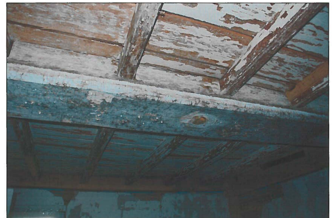
Figure 4: Floor Framing in the Dennis House. Note Wide and Shallow Summer Beam and Chamfered Beam and Joists of this New English, Post-Medieval Type of Box Frame.
