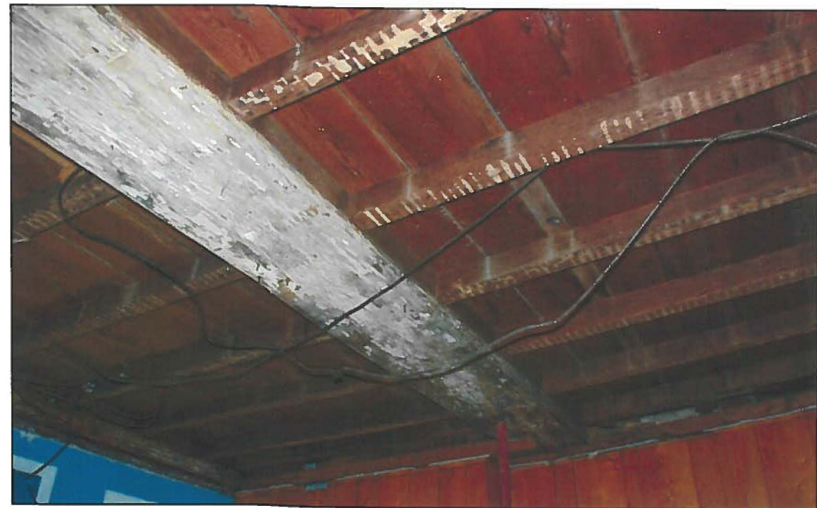
Figure 6: Griffith House Floor Framing, also New English, Post-Medieval in Type. Note Similarity of Wide and Flat Proportion to the One in the Dennis House.
