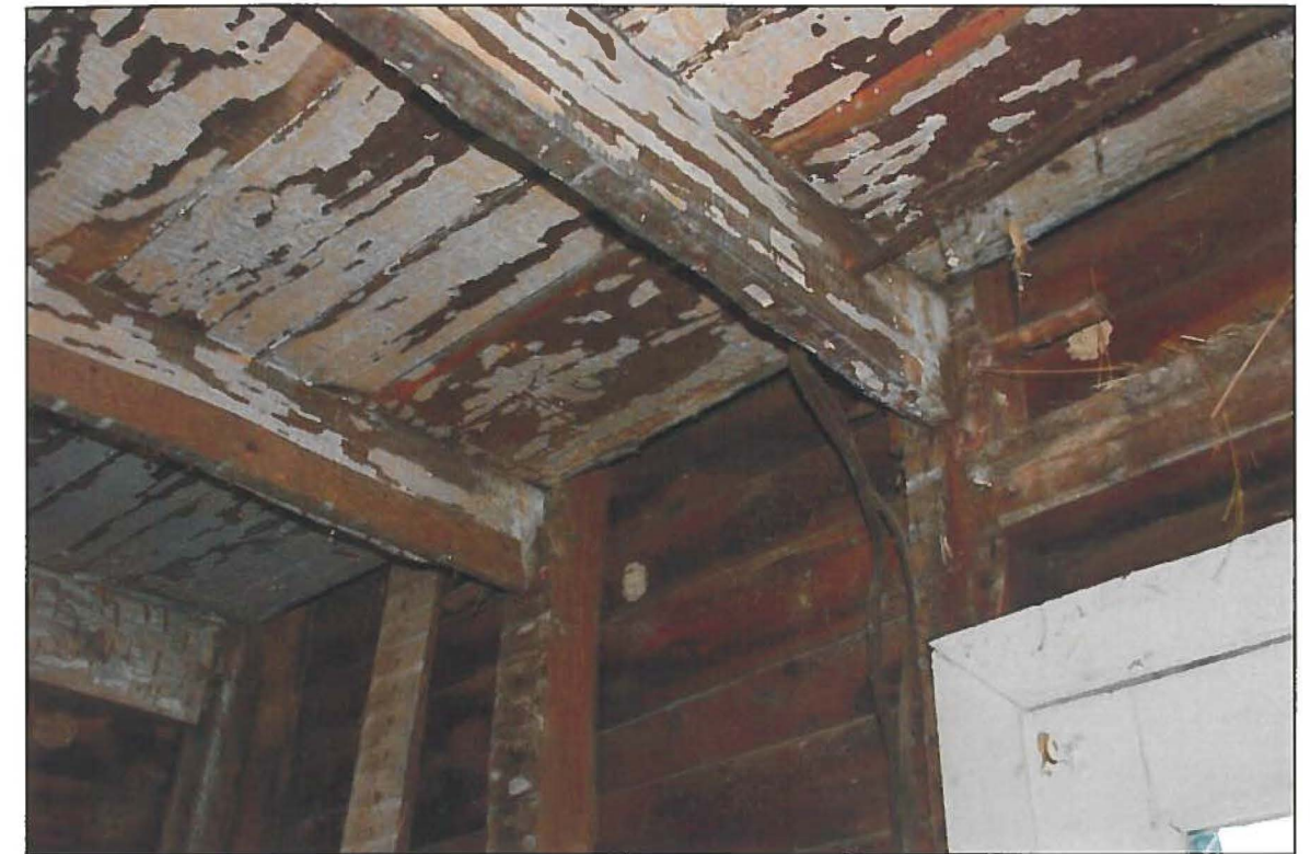
Figure 22: Richman House H-Bent Construction
