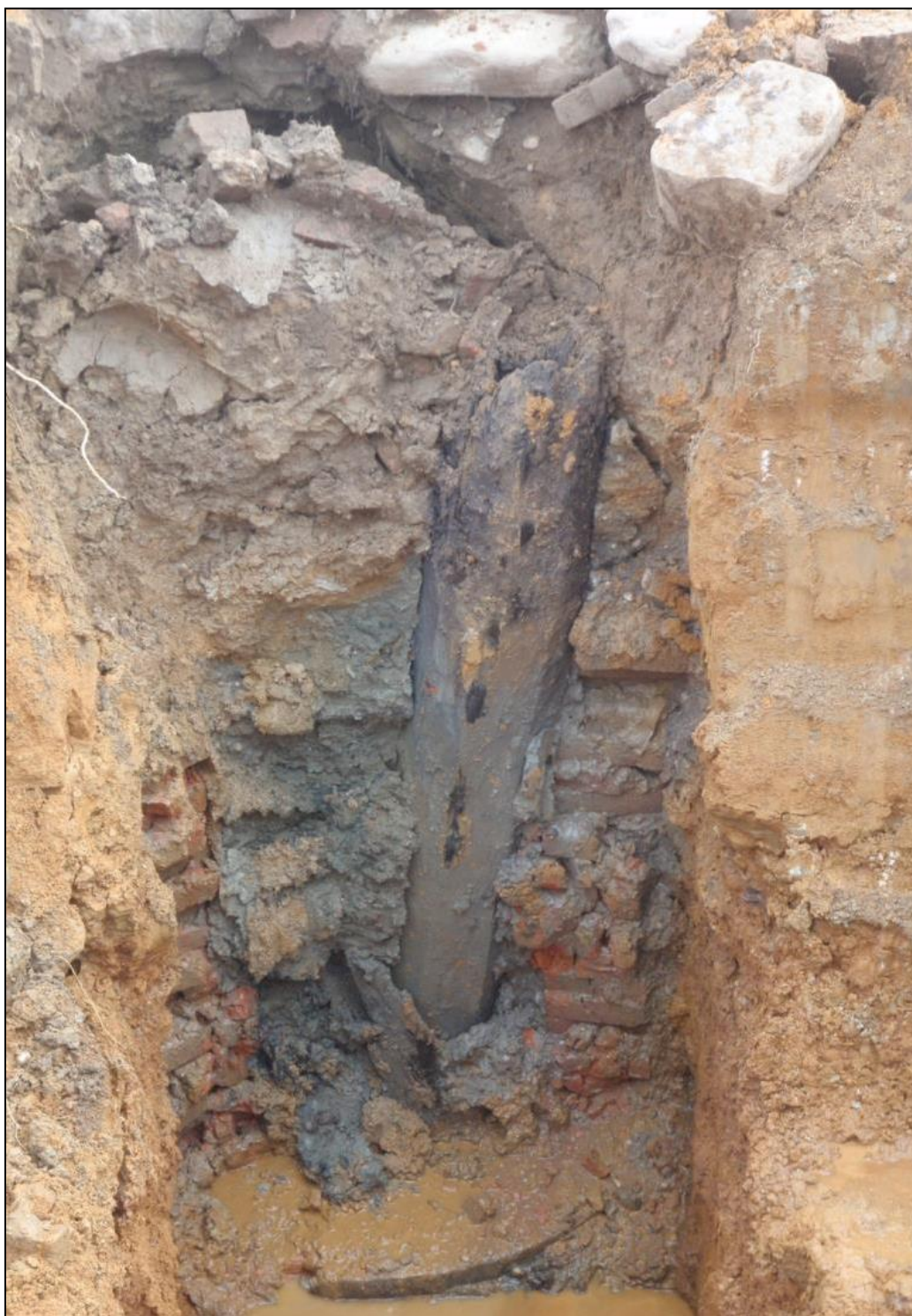
Figure 8: View of the Interior Structure of the Dairy Well Showing the Central Hexagonal Shaft and Circular Pump Base.
